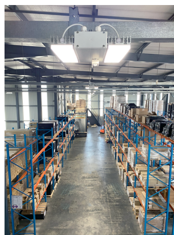
Warehouse installation in the VS building with Blu2Light sensors
