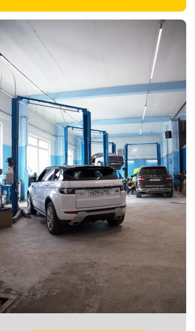
During the reconstruction of Fast Cust Tuning Atelier the objective was to achieve a uniform, cost-effective, affordable and highquality lighting to replace the old lighting fixtures with fluorescent lamps. The large ceiling height complicated quick replacement of failed lamps. Therefore, new lighting was carried out using LED lighting fixtures.
